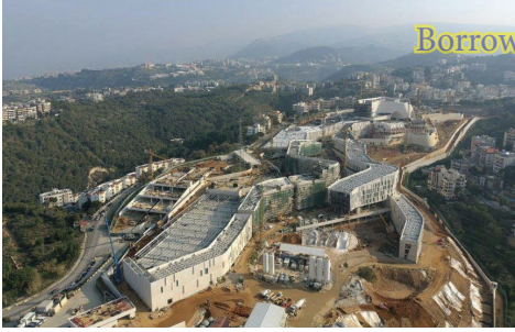
U.S. embassy complex under construction in Beirut. [Source: edition.cnn.com]
