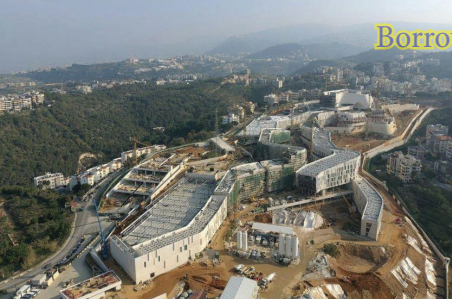
U.S. embassy complex under construction in Beirut. [Source: edition.cnn.com]
